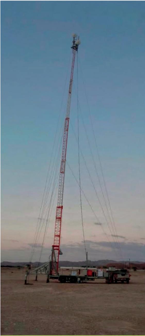
Solar Powered Radio Tower
